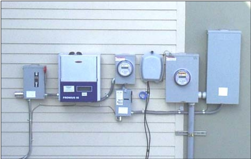
Example of components used to tie into your standard power grid. These will be added (l to r): 1. DC Disconnect 2. Inverter 3. PV Meter 4. AC Disconnect These are pre-existing on your home: 1. Cable/phone box (perhaps) 2. Revenue Meter 3. Breaker Box, or Load Center
