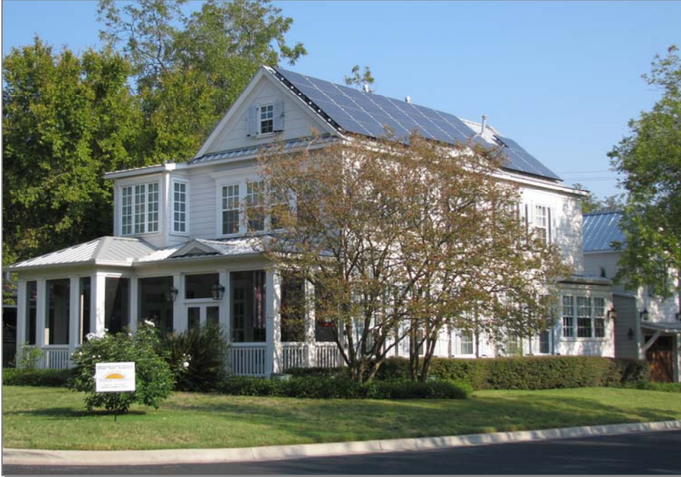
Example of a 6kW system consisting of 30 panels at 200 Watts each.
